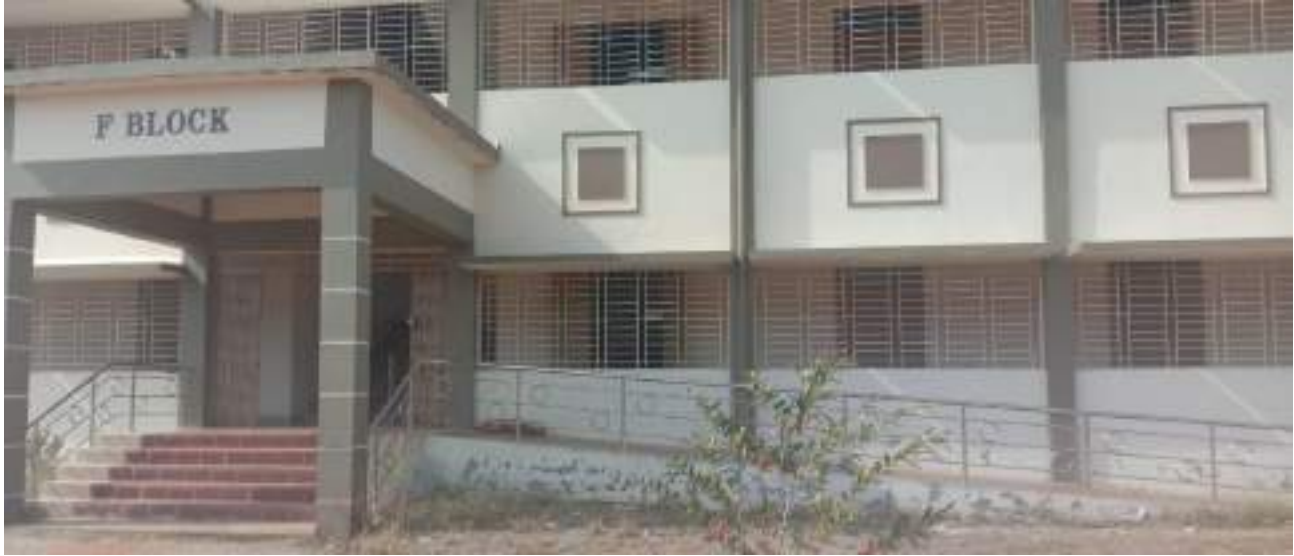
RAMP IN F BLOCK
