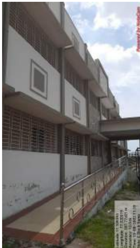
RAMP IN E BLOCK
