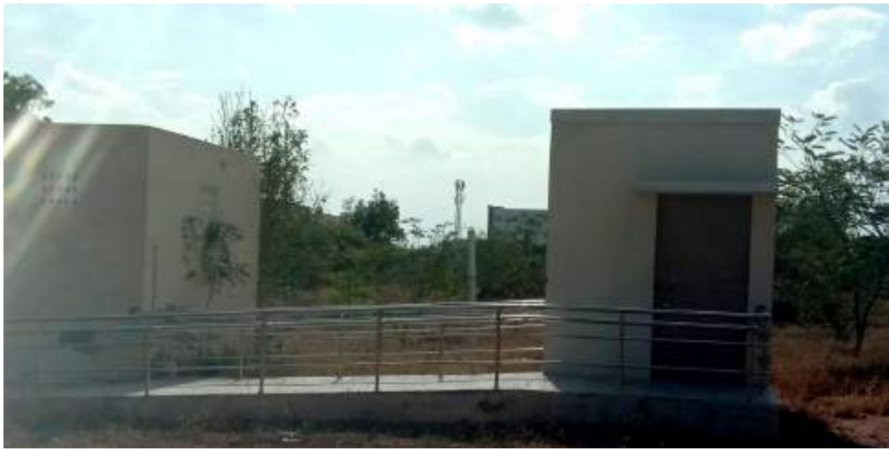
Ramp in F block Rest Room
